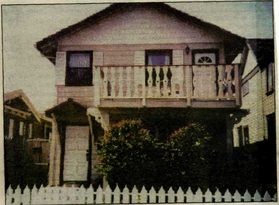
Santa Cruz plans to demolish perfectly habitable Beach Flats homes like this to make way for a new roller coaster at the Boardwalk.
