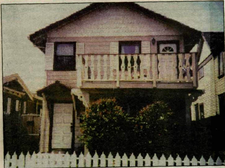
Santa Cruz plans to demolish perfectly habitable Beach Flats homes like this to make way for a new roller coaster at the Boardwalk.
